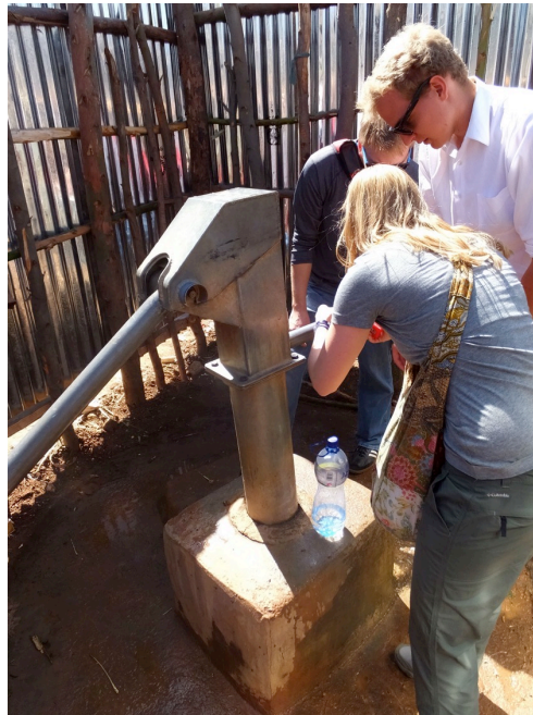
Well # 2 30 m, almost dry
