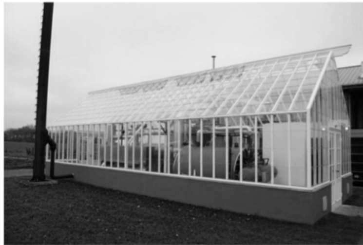
Fig. 5. Biochar plant in Denmark, with 35 KWe cogeneration capacity, powered by Stirling engine.
