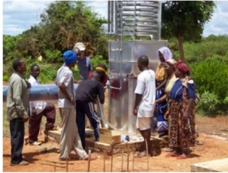
Figure 2. Local people helped install the solar icemakers.
