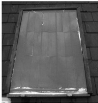
Figure 4-7 A home-made clip fin collector.
