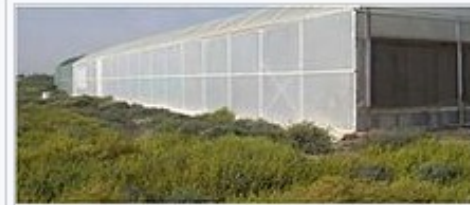
Figure 4. Two years into operation from the back of the greenhouse
