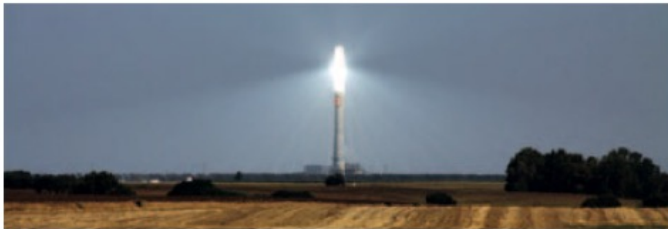
Photo 3.1 The Gemasolar power tower near Sevilla (Spain)
