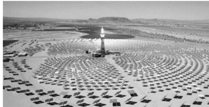
FIGURE 10.6 Photograph of the Solar Two central receiver plant (source: www.energylan.sandia.gov/sunlab/Snapshot/STFUTURE.HTM ).
